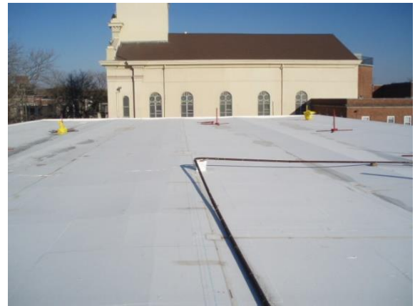
We designed the roof replacement on Polly McCabe School .
