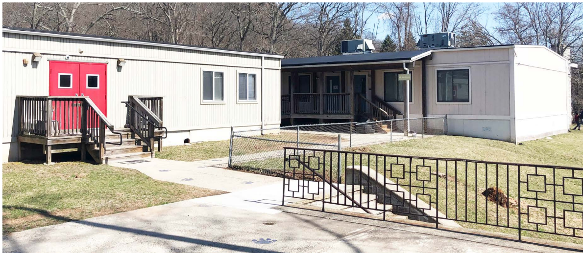
Portables for classrooms at West Rock Elementary
