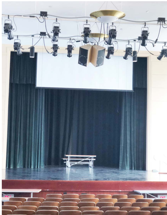
Stage lighting at Hooker Elementary that has never functioned
